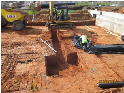
Sumps and drainage started under new swimming pool
