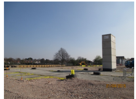
Foundations and stone filling complete to main building area
