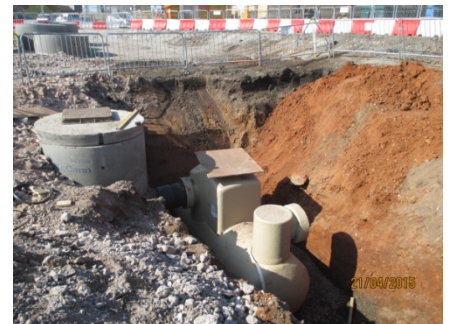
Deep drainage started with the car park petrol interceptor being installed
