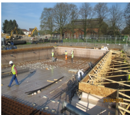
Main swimming pool taking shape
