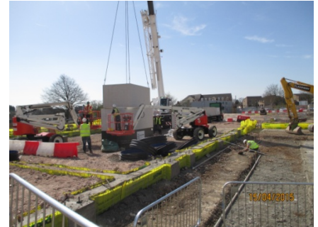
Precast concrete lift shafts being erected
